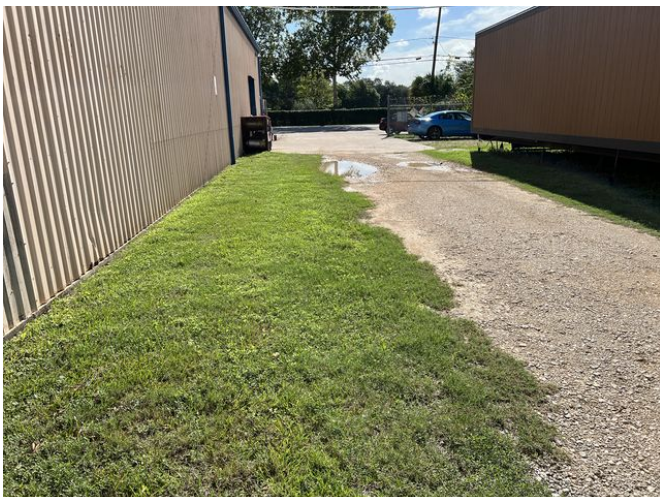
Standing water front delivery well
