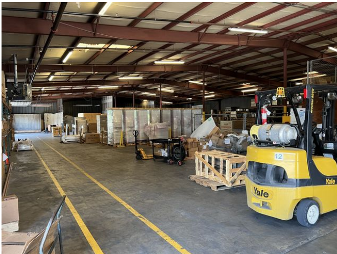
Building is steel frame construction on slab
