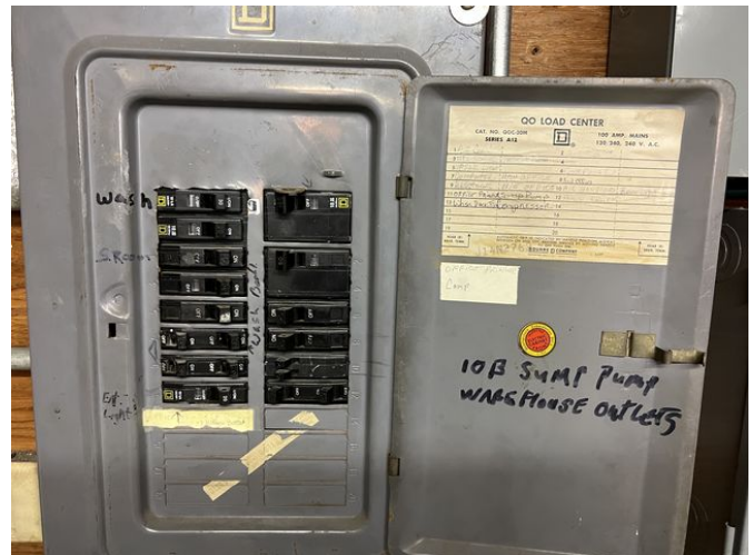
Labels missing at dead front cover
