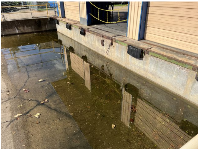
Standing water front delivery well
