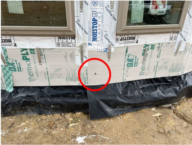
Hole T-ply rear master bedroom wall
