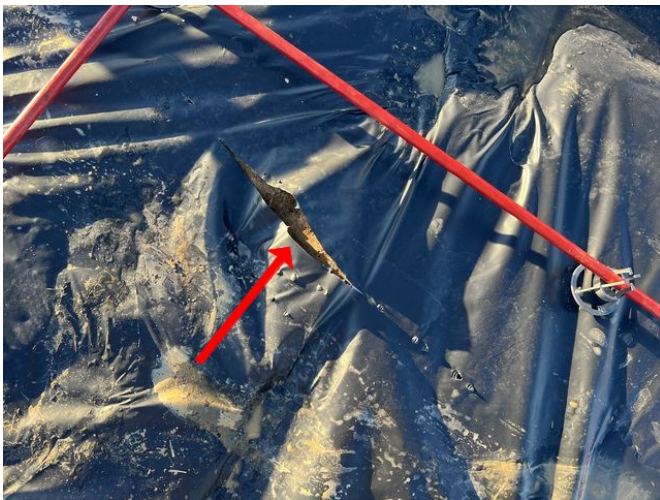
Tear vapor barrier interior pad near front porch
