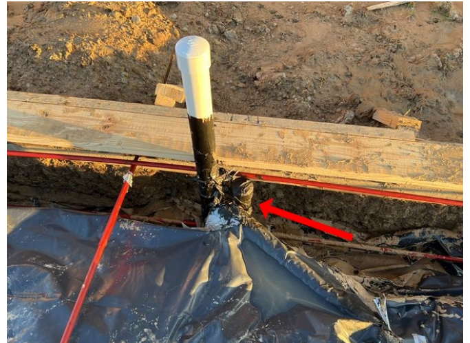
Capped drain pipe at right perimeter beam
