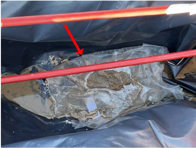
Remove construction debris from footings
