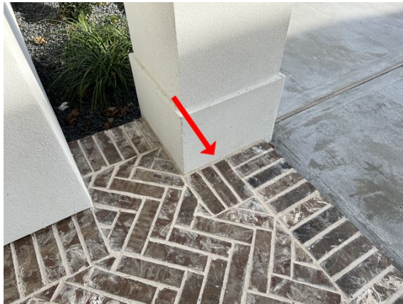
Stucco clearance front porch columns
