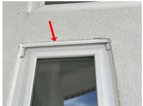
Z-flash drainage plane caulked above windows
