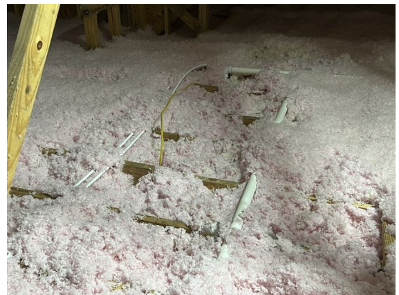
Redistribute insulation where moved at attic
