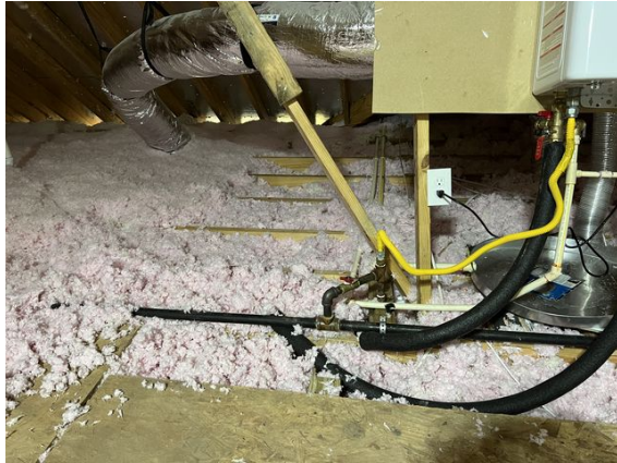
Redistribute insulation where moved at attic
