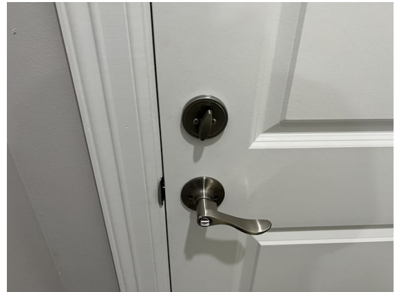
Lock and latch not aligned garage entry door
