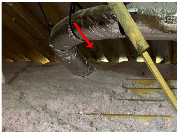
Attic mechanical fan not positioned over hole
