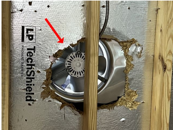
Attic mechanical fan not positioned over hole
