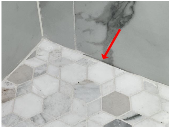
Caulk master shower enclosure
