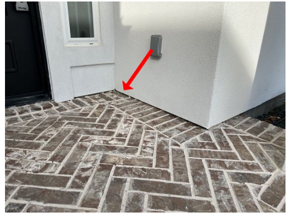
Stucco clearance front porch walls
