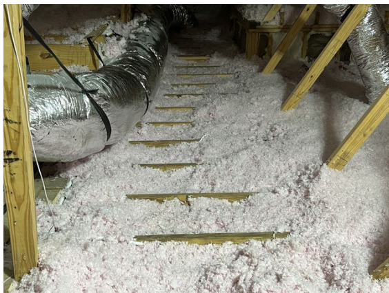
Redistribute insulation where moved at attic
