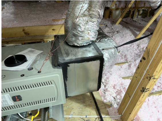
No fresh air intake at A/C return
