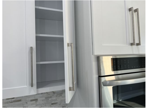
Kitchen cabinet door binding at oven
