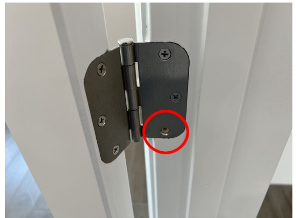
Hinge fasteners missing office door
