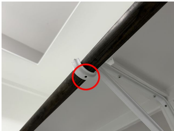
Clothes rods not secured rear guest bed closet
