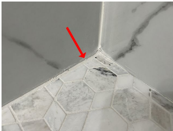
Caulk front guest bathroom shower enclosure
