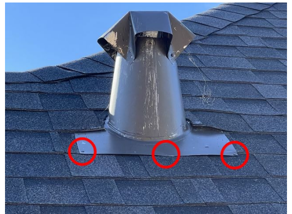
Caulk face nailed roof jacks
