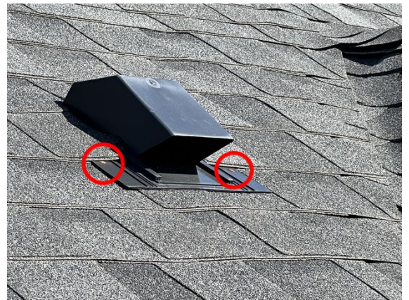
Caulk face nailed roof jacks
