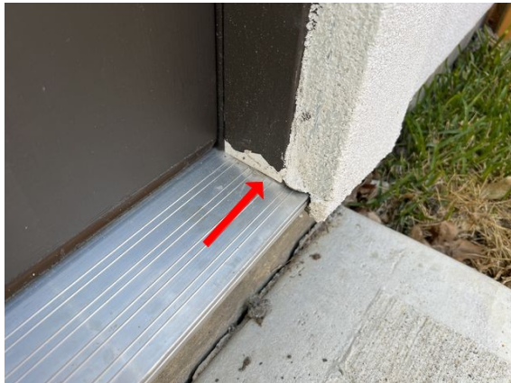
Threshold not caulked left garage door
