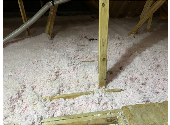
Redistribute insulation where moved at attic
